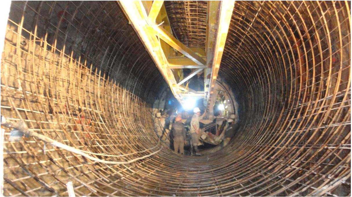
Headrace Tunnel – Rebar Fixing
