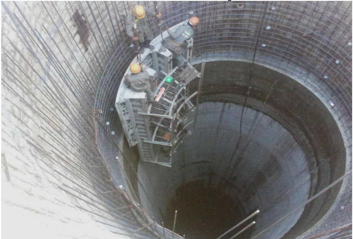
Surge Tank – Formwork Installation for Lining Concrete
