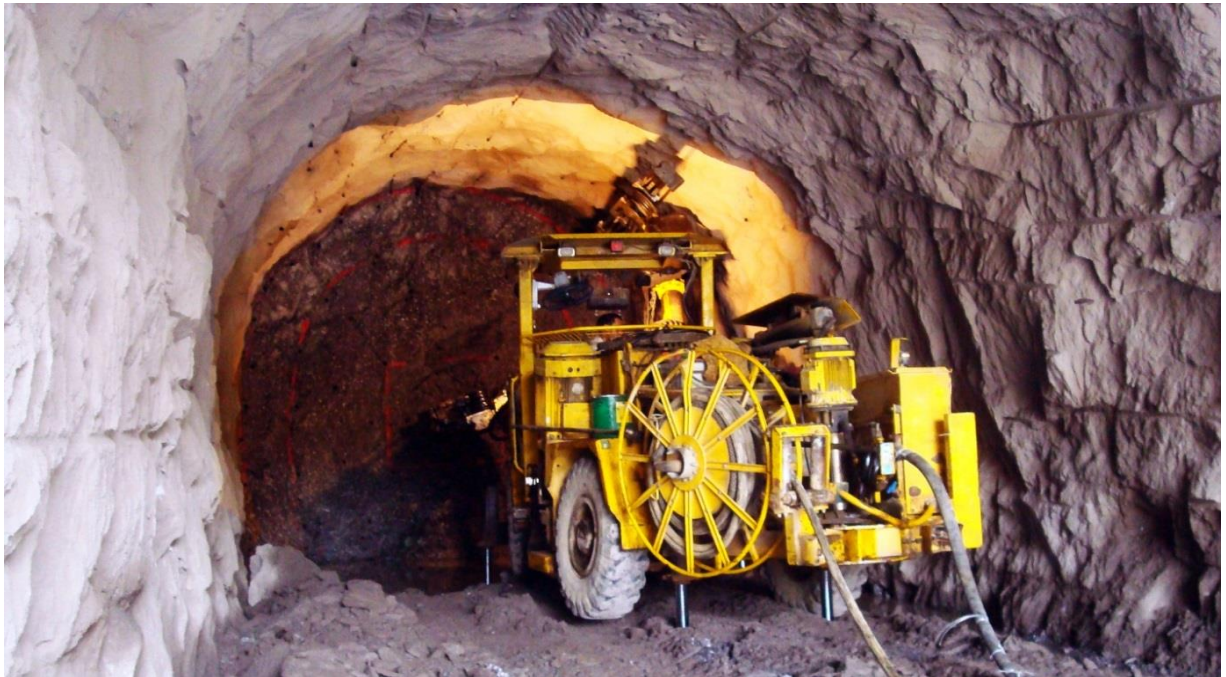
Headrace Tunnel Excavation
